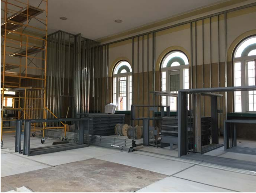
Steel in the future library site
