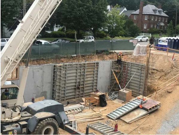
Concrete work in the cafeteria
