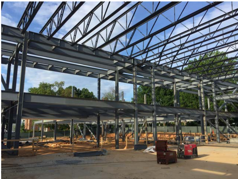
Steel erection in the gym
